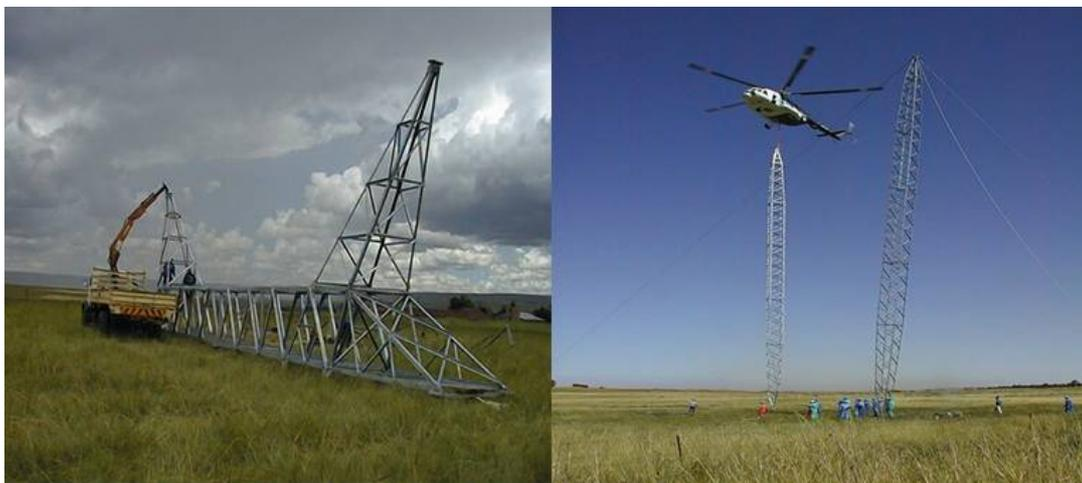
**Figure 3.14:** Assembly and Erection of towers (Step 12)
